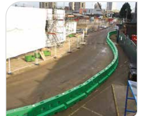
Forming bend around site perimeter
