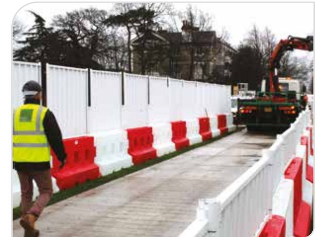
Full & half hoarding securing site entrance
