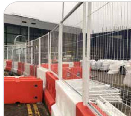
GB2's with fence securing building materials
