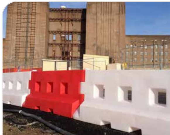
GB2's securing large demolition site
