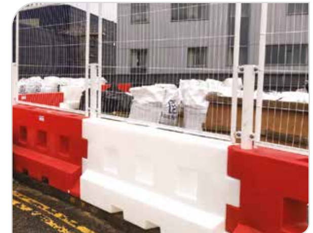
GB2's on site with mesh fence
