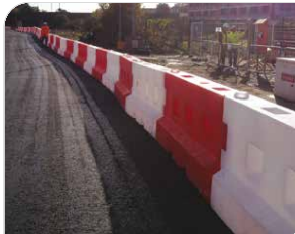
GB2's forming road perimeter on site
